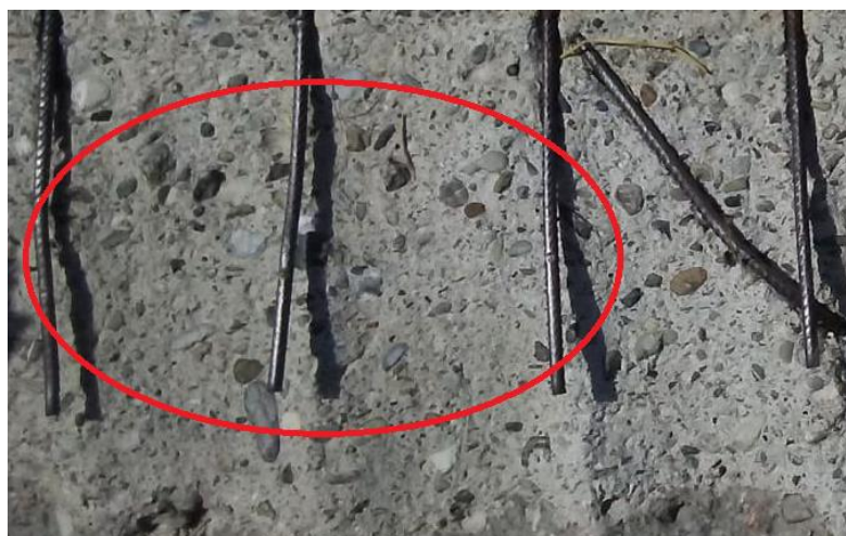
Fig.3.1 – Armature in alveo abrase.
